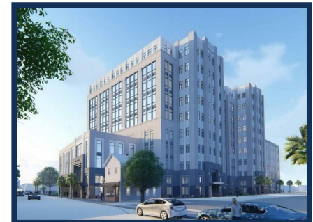
FREIGHT YARD STATION 82 Mary Street 120,000 SF | 9 Stories Structured Parking Developer: Cobalt Properties Status: Final BAR Approval
