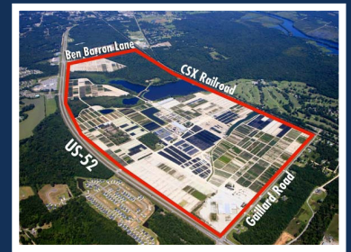
739 GAILLARD ROAD A&R Logistics leased 615,000 SF.
