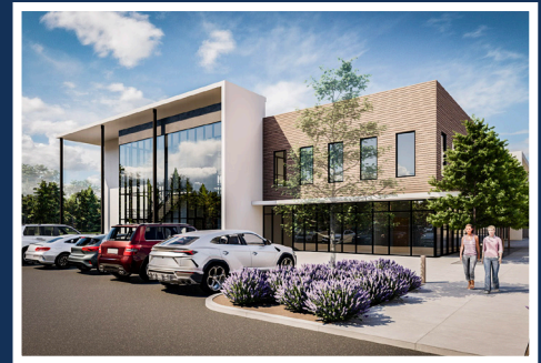
THE HUB @ NEXTON BUILDING 2 Q4 2023 DELIVERY
