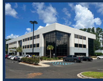
FABER CROSSING North Charleston 10,000 SF Available
